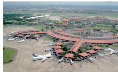
Indonesia Airport Control System
