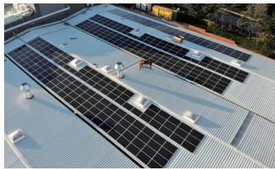
Bulgaria Industrial&Commercial Energy Storage System
